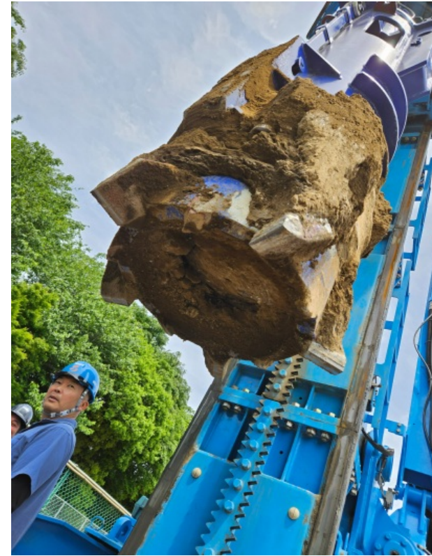
Take pile away
