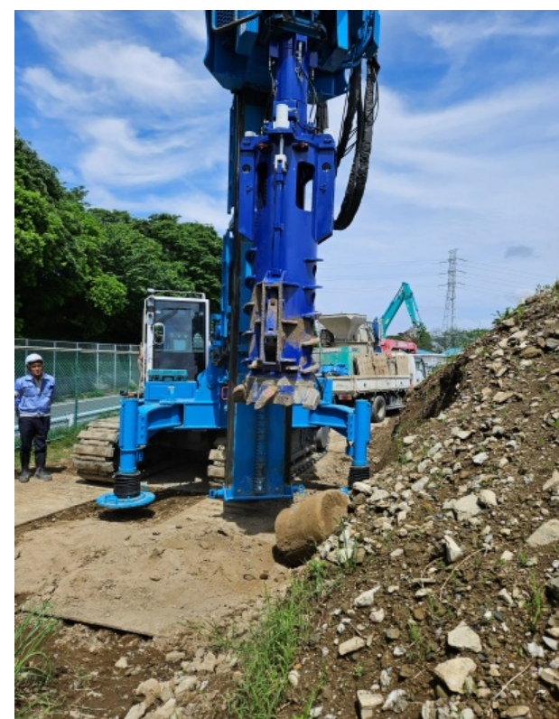
Drop off pile
