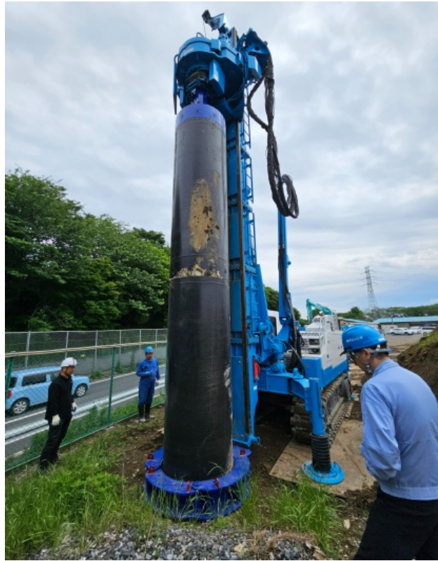
Installation of casing
